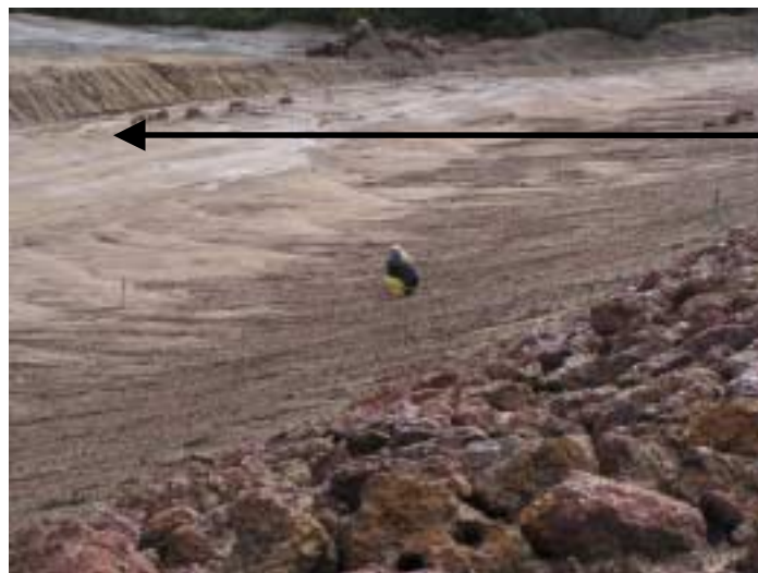
Perimeter drain set well back from the toe of the slope
