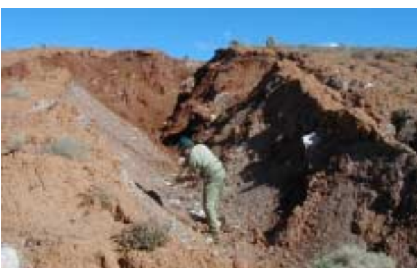
Tunnel collapsed to form a gully
