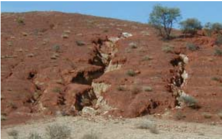
Gullies associated with berm overtopping
