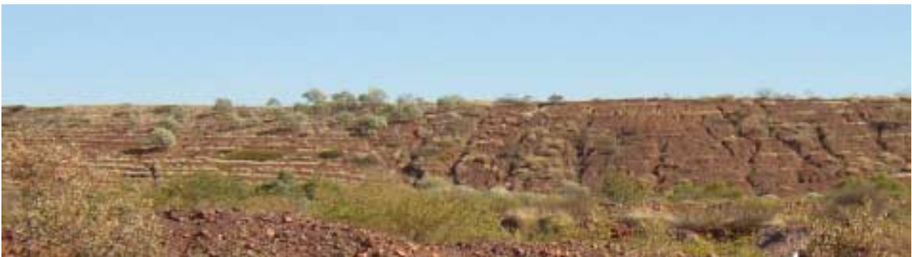
Waste dump with small rip lines and little erosion on left, large rip lines and gullies on right.
