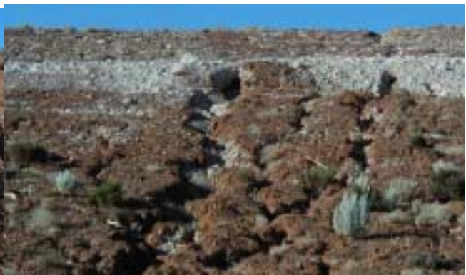
Tunnelling through a berm
