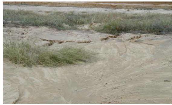
Sediment deposition in a berm 12 months after completion of rehabilitation, and flow already overtopping the berm
