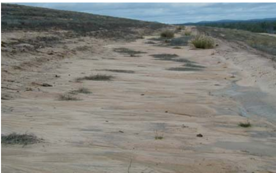
Sediment deposition in a berm 12 months after completion of rehabilitation, and flow already overtopping the berm
