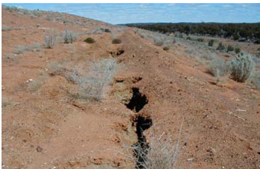
Development of tunnel erosion in a level berm due to ponding of water, leaching of salt, and increase in clay dispersion. Ponding is a strong driver of tunnelling, even on some non-dispersive spoils.
